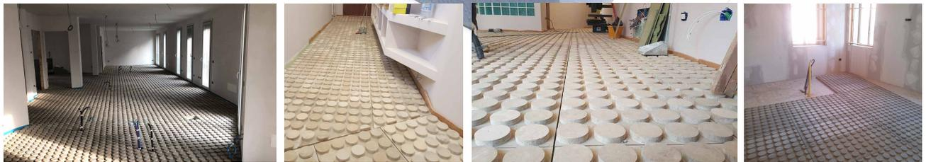
BETONRADIANT IS A MODULAR SYSTEM FOR TRADITIONAL AND ELEVATED DRY FLOOR RADIANT HEATING SYSTEMS, FLOATING FLOORS ON LOOSE MATERIAL OR OVER HEIGHT-ADJUSTABLE SUPPORTS.
